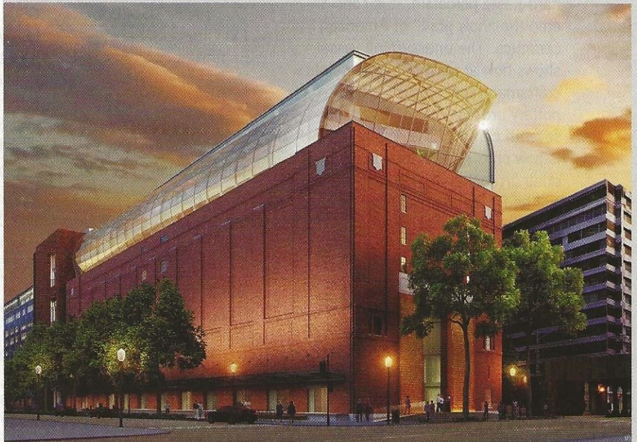
Two floors were added to the historic Terminal Refrigerating and Warehousing Co. building to house a 470-seat performing arts center and a 500-seat “gathering room” for events at the Museum of the Bible.
