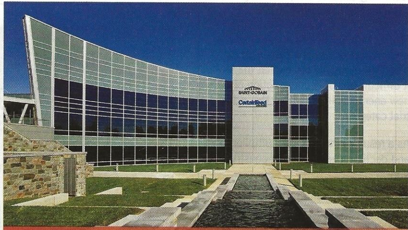
The west and south facades of Saint-Gobain’s U.S. headquarters in Malvern, Pennsylvania, feature 17,000 square feet of SageGlass, marking one of the largest installations of electrochromic glass to date.
